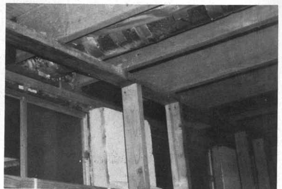
Insulation of duct and overhang, part of Princeton retrofit package C.
