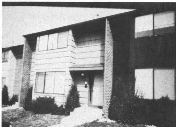
Front view of Quad II townhouse rented by Princeton. Masonry firewalls project beyond the structure in brick. Central projection (with windows of living room and master bedroom) terminates one foot above ground level (behind bushes).
