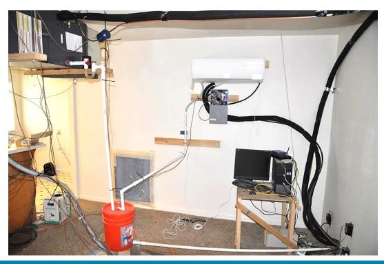
FIGURE 9. WALL-MOUNTED VCHP FAN COIL AND REFERENCE SYSTEM AIR HANDLER AT GRANGE HOUSE
