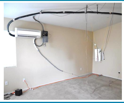
FIGURE 11. WALL-MOUNTED VCHP FAN COIL AT CALEB HOUSE (1 OF 3) & SUSPENDED, SHIELDED SENSORS
