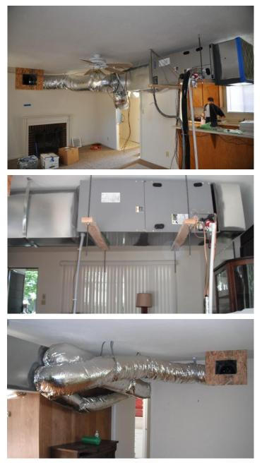
FIGURE 6. TYPICAL REFERENCE HEAT PUMP SYSTEM INSTALLATION WITHIN CONDITIONED SPACE
