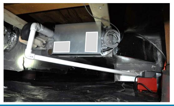
FIGURE 10. CRAWLSPACE-MOUNTED VCHP DUCTED AIR HANDLER AT MAYFAIR HOUSE
